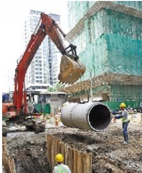
Figure 7 Underground drainage system will be improved including the increase of the number of drainage pipes as well as the length of the pipes
